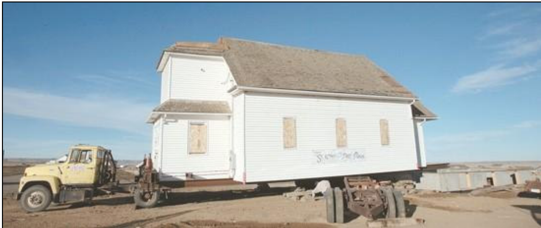
Workers prepare to move Faith Lutheran Church onto its new foundation.
